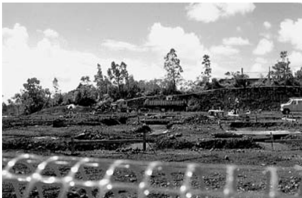
Figure 2. Hilo Base Facility construction, September 1997.
